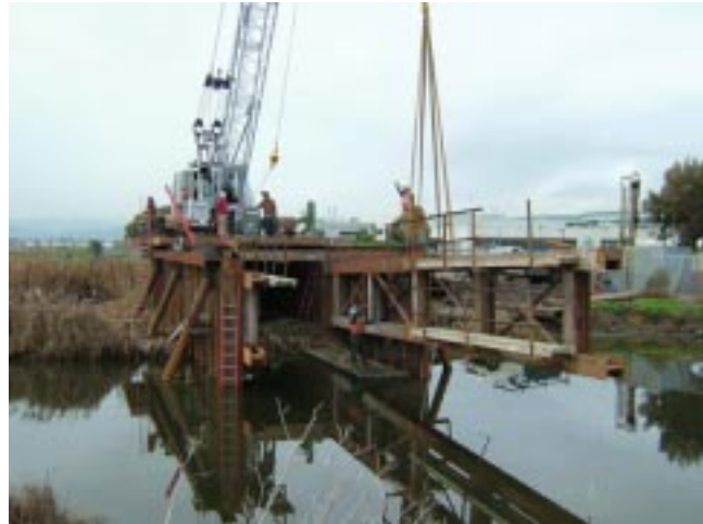
A picture from the early construction.
