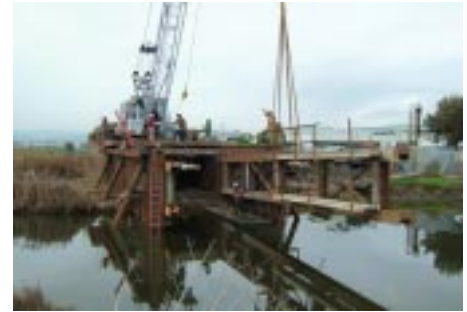
Photo: an early construction photo
