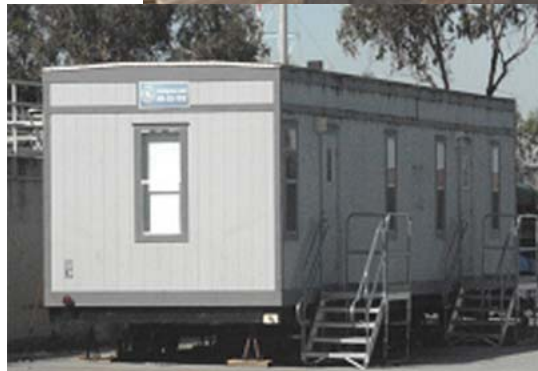
Staff offices in temporary trailers
